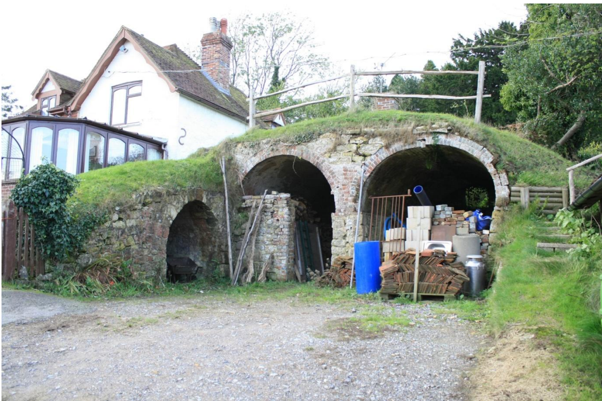
Plate 20. Curious structure built to the south of the barn, function unknown but potentially for lime burning.
