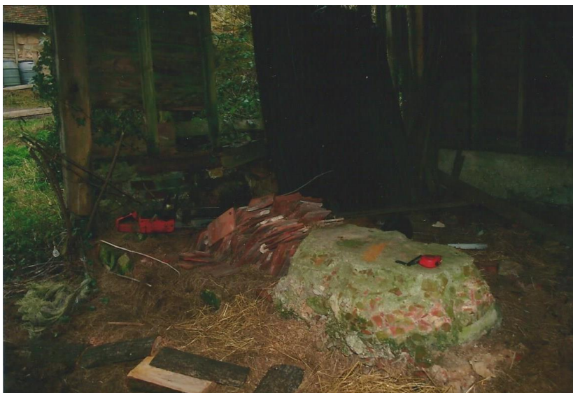
Plate 29 Before renovating inside looking south (Reproduced by kind permission of Jamie French)
