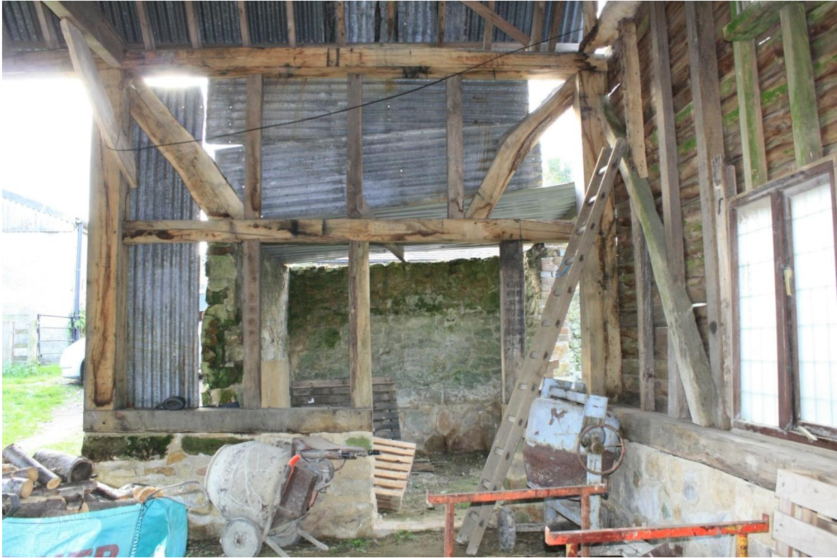
Plate 13 Re-built south elevation between truss A and B
