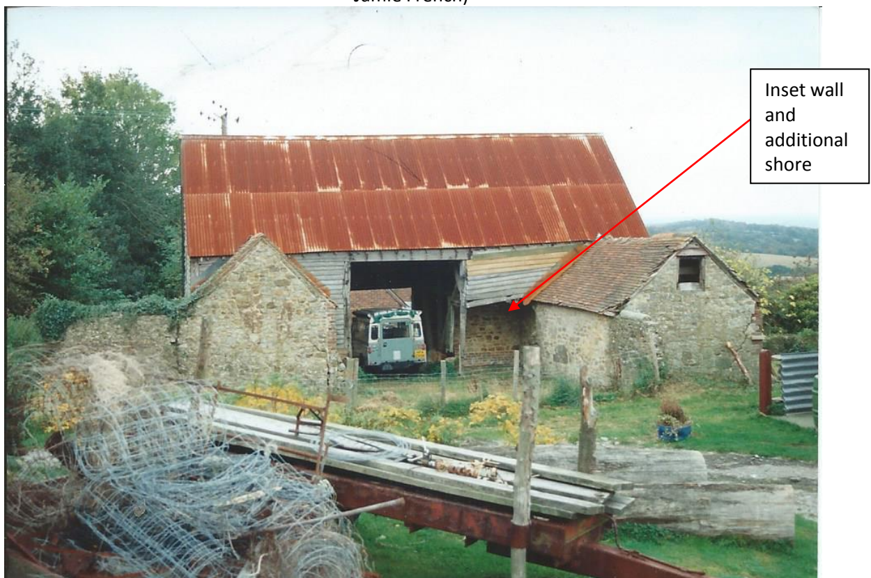
Plate 35 Before renovating looking towards the south elevation (Reproduced by kind permission of Jamie French)
