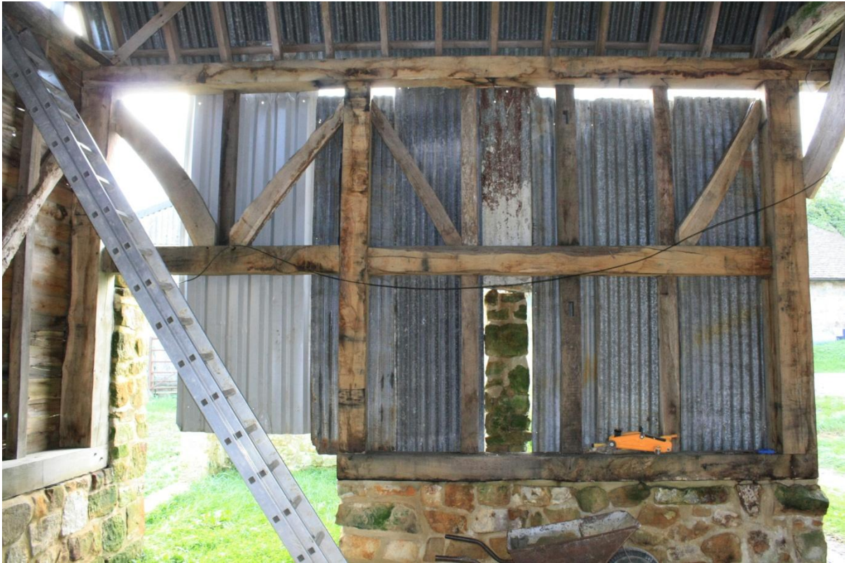
Plate 14 Re-built elevation between truss C and D
