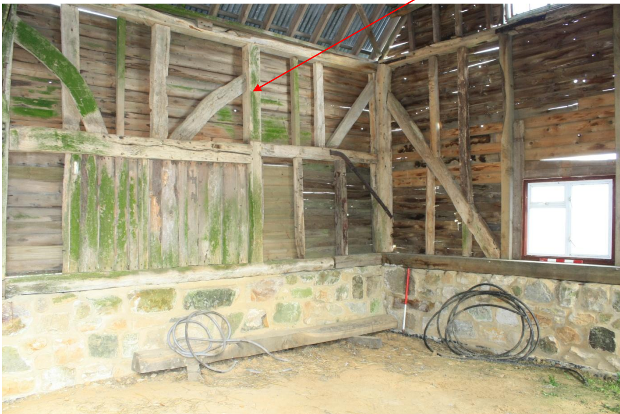
Plate 12 north elevation between truss C and D (scales 1m and 50cm)
