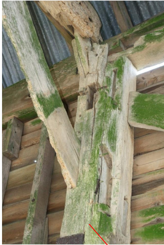
Plate 6 and 7 truss C principal post
