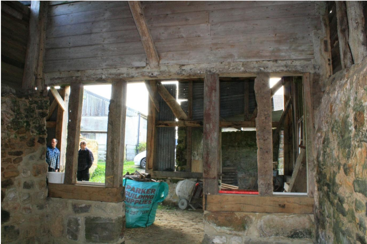
Plate 19 The replaced plinth and sole plate of the north west outshot
