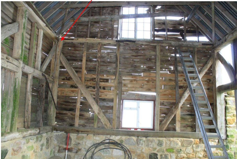
Plate 8 and 9 Truss D and the principal post
